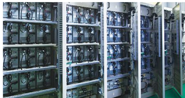
2. Lithium-ion capacitors are effective for addressing short-cycle frequency fluctuations. (Courtesy of Hitachi)
